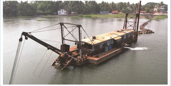
OPERATION OF DREDGER
