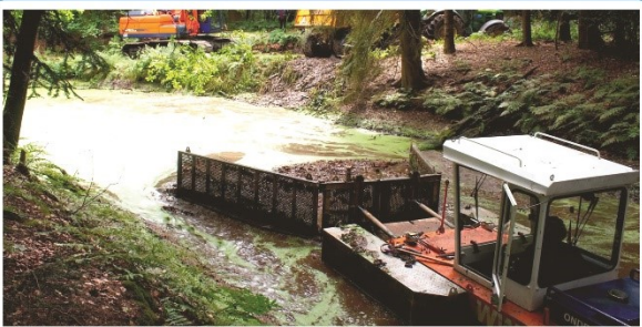
OPERATION OF SILT PUSHER
